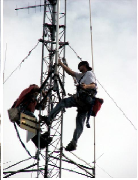
Work being done on Larry's tower, KA9KDC, this past Tuesday afternoon by Tower Works (a commercial tower company). This work was necessitated after tornado that plowed through Wheaton on the Afternoon of August 23rd. Left picture shows the clubs 2M antenna being realigned to the vertical position. Work also performed by Tower included replacement of guy and structural hw. See the pictures in last month's Hamletter to note the differences.
